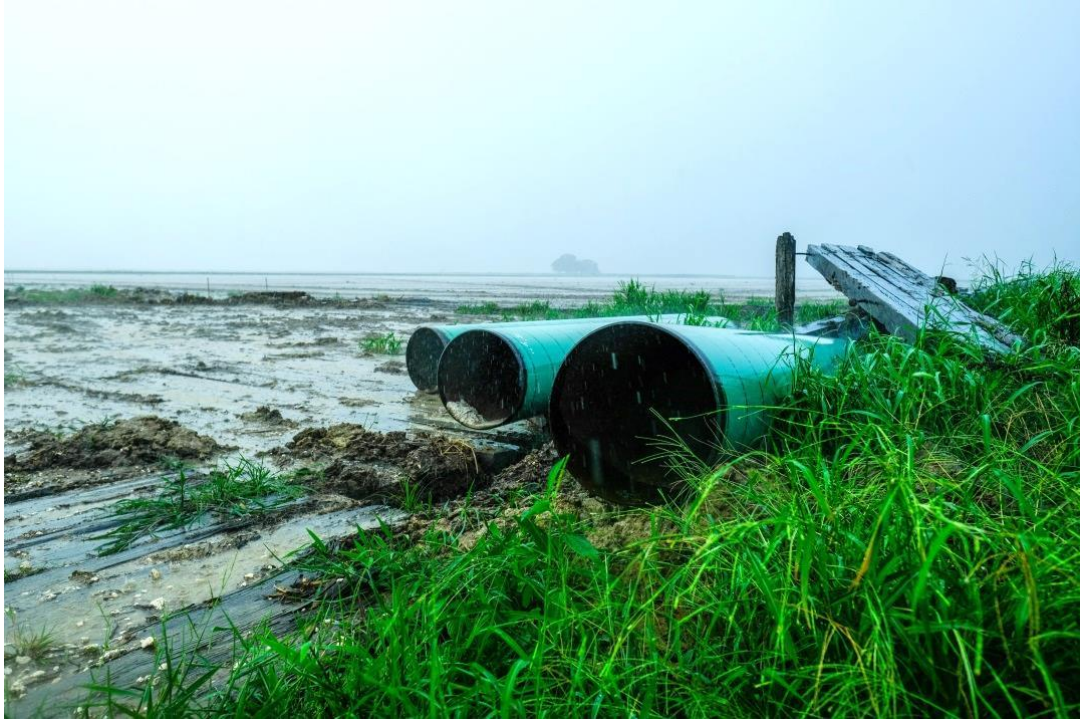
Caption: Excess pieces of pipe for the Bayou Bridge Pipeline in the southwest prairielands, west of L'eau Est La Vie
