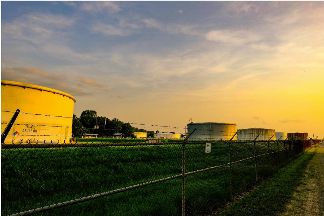
Caption: Weathered crude oil storage tanks fenced off on privatized land, adjacent to the St. James neighborhood of Burton Lane; the precise region of the Bayou Bridge Pipelines terminus where its oil will be exported to local industry
