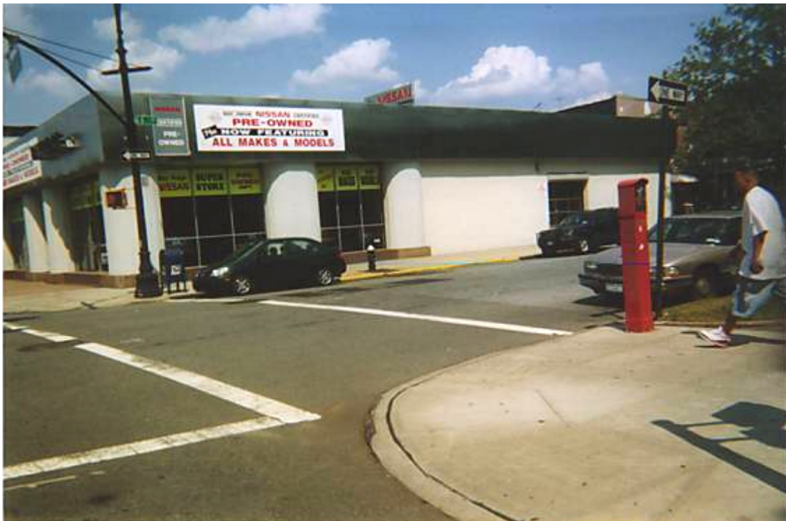
In 2007 the building still stands but is now home to a car dealership. Photo: George Hansen (2007)
