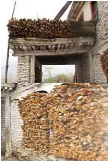
Plate: 4.13 Stored wood
