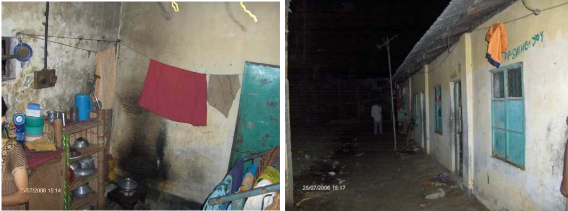
One storey mess building shared room housing
