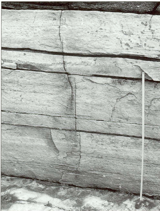
Fig. 2. Linking up of extension fractures in gneiss on the island of Øygarden (Toftøy). View northeast; the fracture aperture tends to increase when meeting with the horizontal exfoliation fractures, at the contacts with the dark amphibolite layers. The steel tape is 1 m long.
