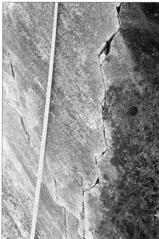
Fig. 6. Extension fractures linked up through transverse shear fractures, modelled in Figs. 7-8. View NNE; the length of the steel tape is 0.8 m.
