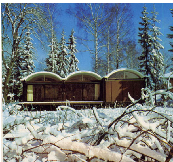
Fig. 47. Sun House, Villa Aall, Fredrikstad
