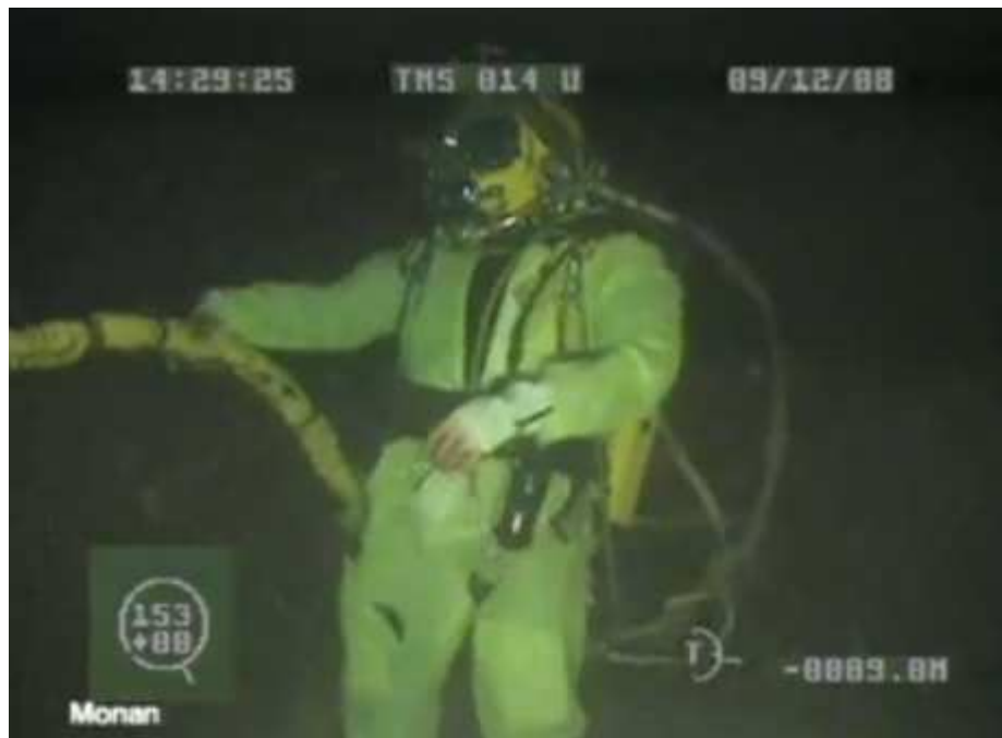
Figure 2. Saturation diver holding his umbilical cable in the North Sea at 89 meters depth.
