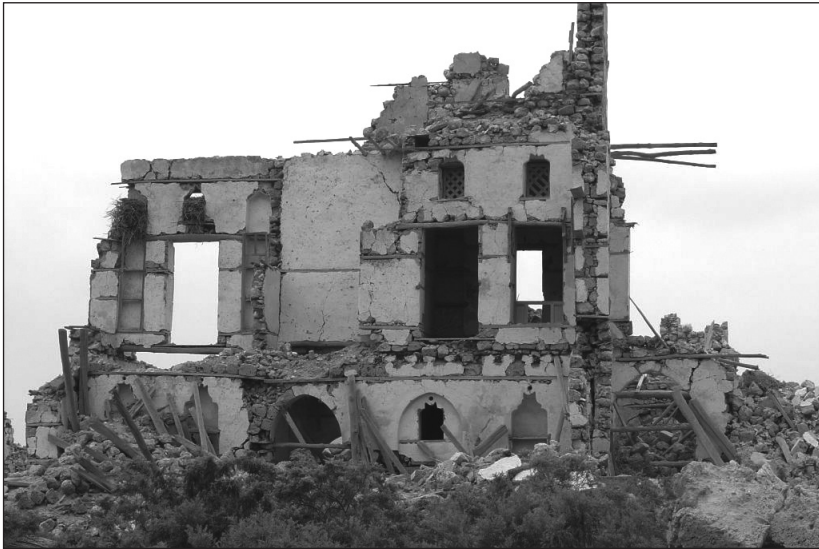
Plate 4.9: Remains of Three Storey-House in Suakin
