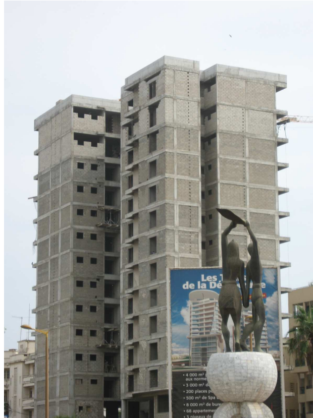
3. Construction project in 'modern' Senegal (Dakar).
