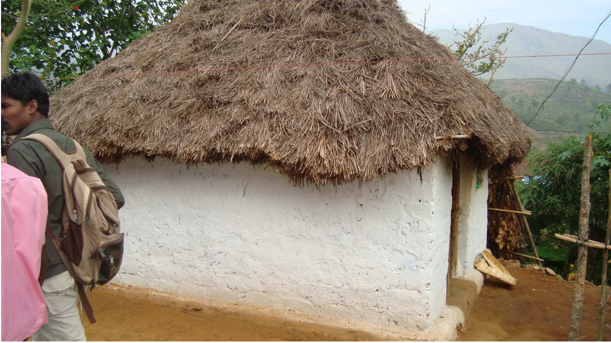
Picture 4.1: Self constructed house of a temporary worker
