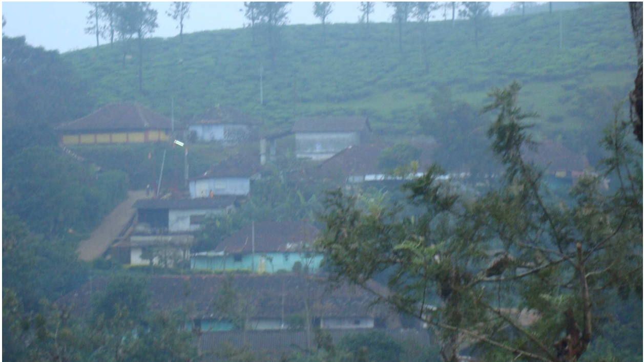
Picture 4.3: Workers Settlement and the Temple (the yellow coloured construction)
