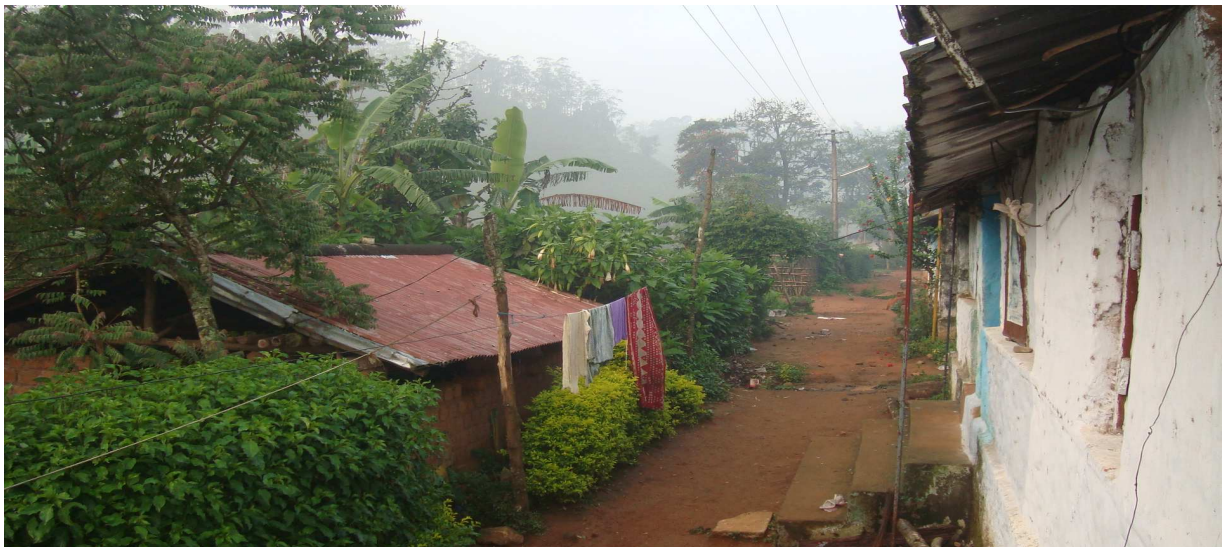
Picture 4.4: Workers' lines (side view)
