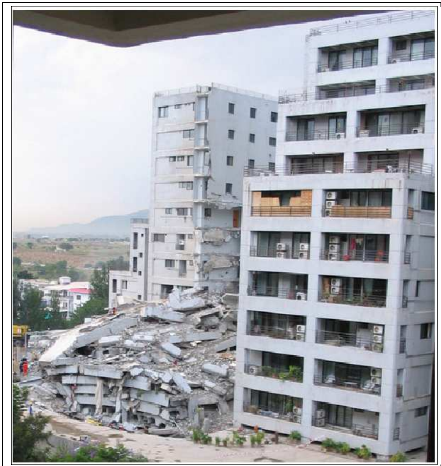
Figure 1.2:- View of collapsed Margalla Tower Islamabad, Pakistan (Google earth).
