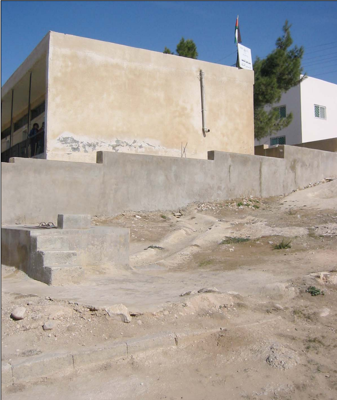
Figure 5.6. Household seven collected rainwater for the roof of the neighbouring school by using a pipe to direct the water to the cistern. This was the cleanest cistern found.
